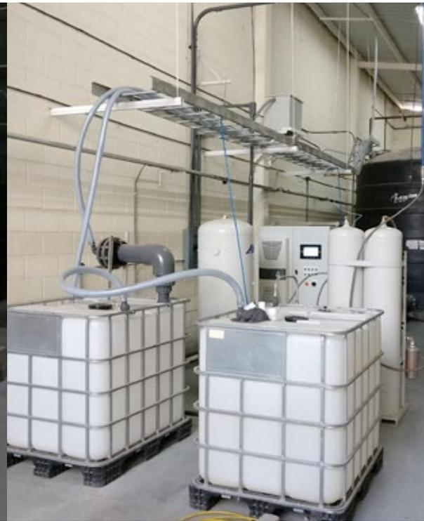
The ozone system is connected to a collection tank for allowing the required reaction time.
