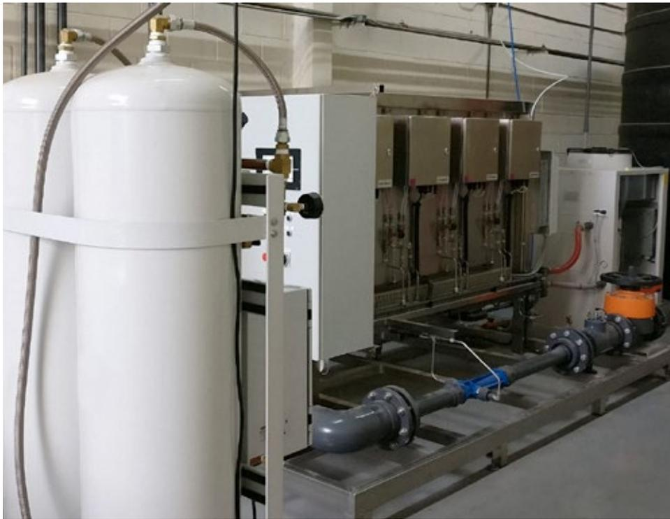
The complete solution designed by Ozonetech, including complete ozone system with optimized ozone dissolution, control unit, oxygen system, cooling unit, reaction tank and foam collection.
